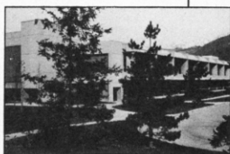
H-P's headquarters in Grenoble.
